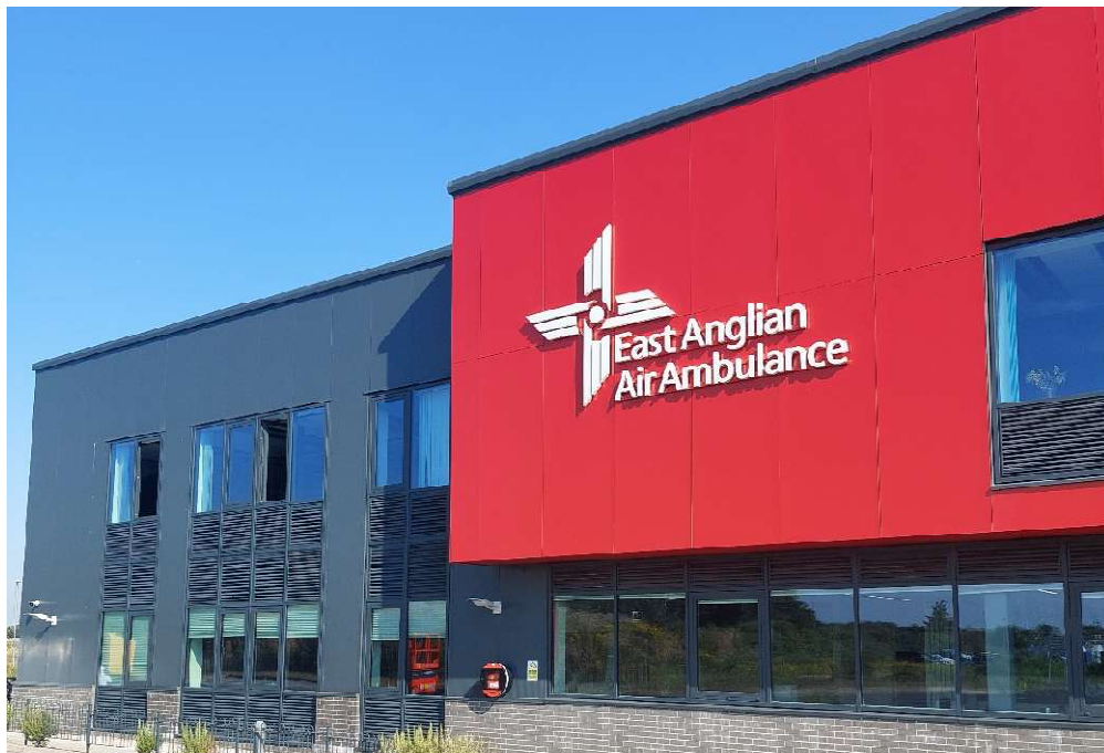
Helimed House, EAAA's Norwich base
